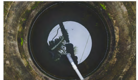
Picture of an uncovered potable water route or pit entrance (manhole).
