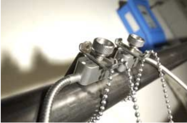
Q3N ultrasonic sensors installed on pipeline
